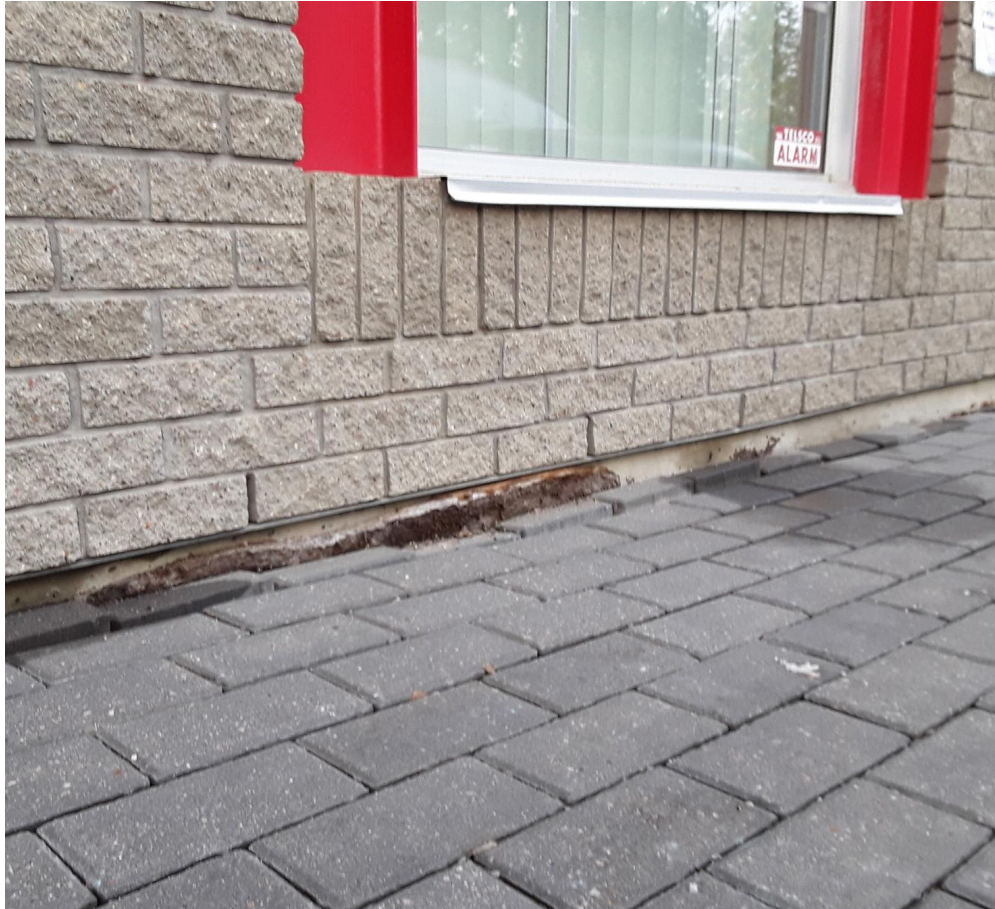
Image: Damaged insulation at exterior wall base.
