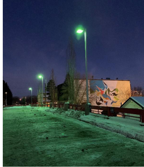
Parking Lot Pole Luminaires (Metal Halide Lamping)
