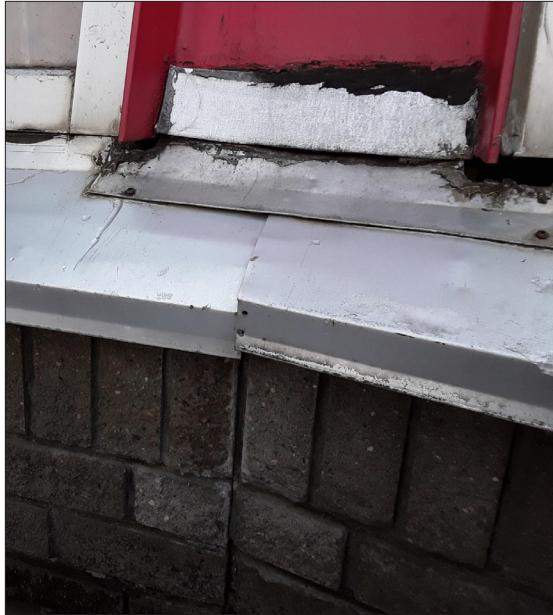
Image: Flashing Damage
