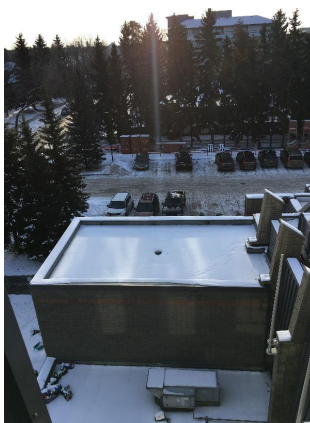
High South Roof
