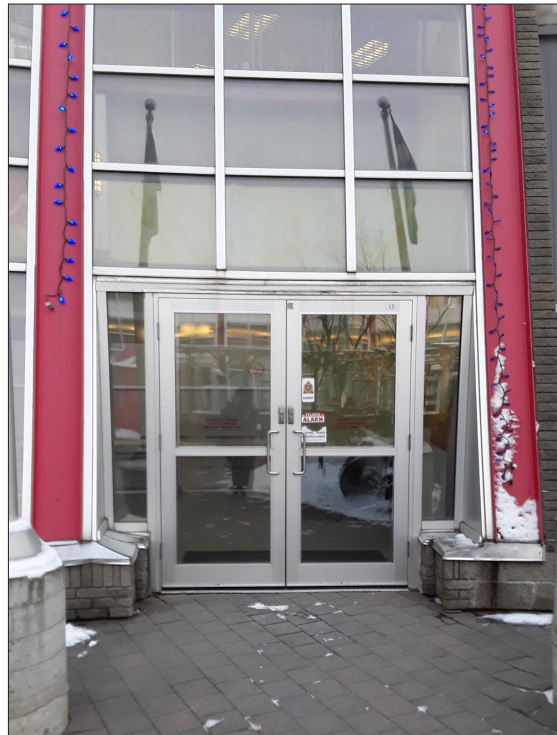
Image: Main Atrium Doors from the Outside
